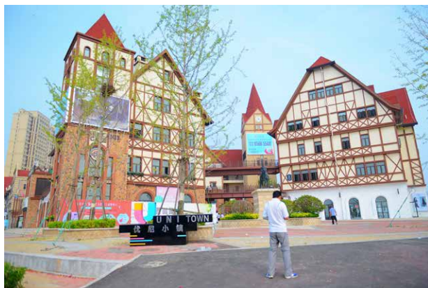
Figure 25: Uni Town, a commercial street, is one of the communities served by the heating and cooling network. Photo credit: City of Qingdao
